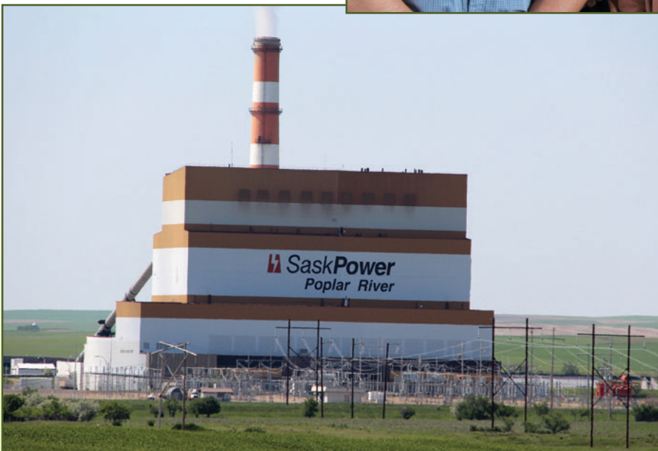
Poplar River Power Plant
